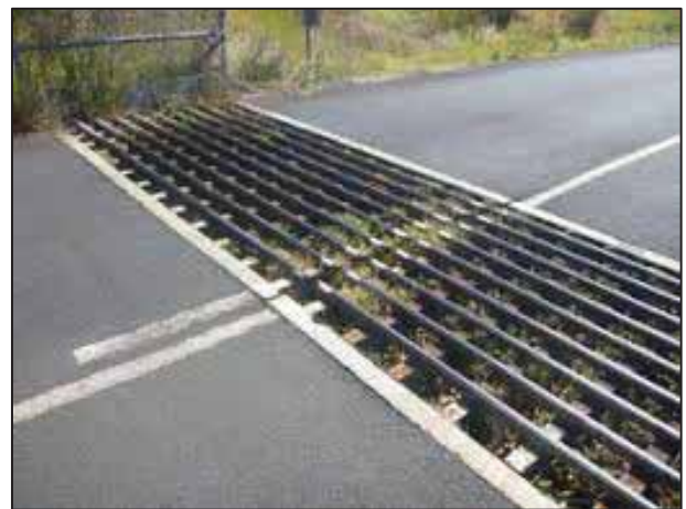
Plate 1 Example of Koala Grid (Source http://www.rms.nsw.gov.au/projects/northern-nsw/koala-grids/index.html )
