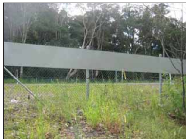
Plate 4 Example of scratch plate at top of fencing (Source https://fencescape.com.au/wildlife-fencing/ )
